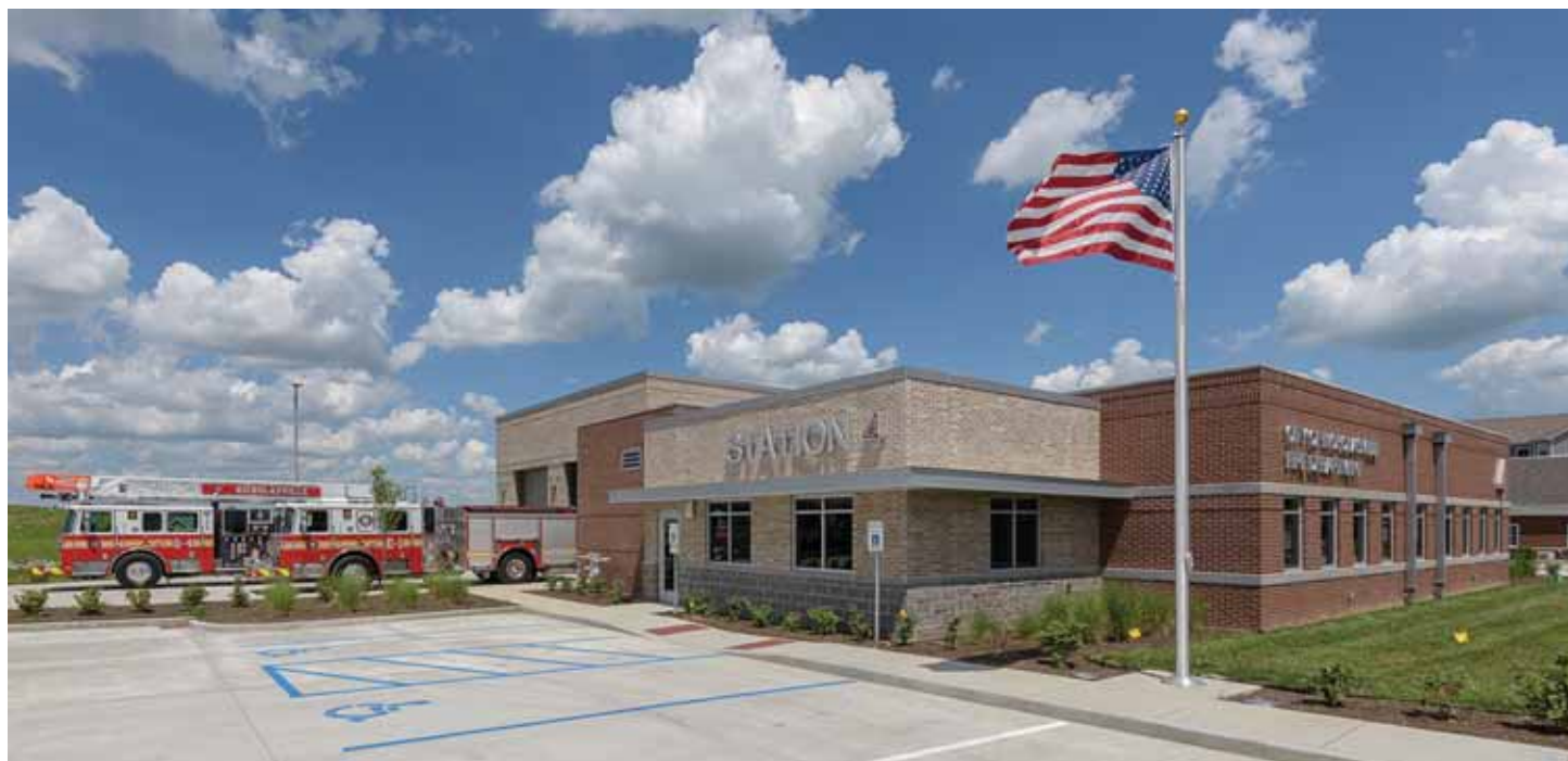
Station 4 opened in 2020 with little fanfare due to COVID-19, but public engagement will resume as soon as it is safe. Photographs provided by Walt Roycraft Photography.
