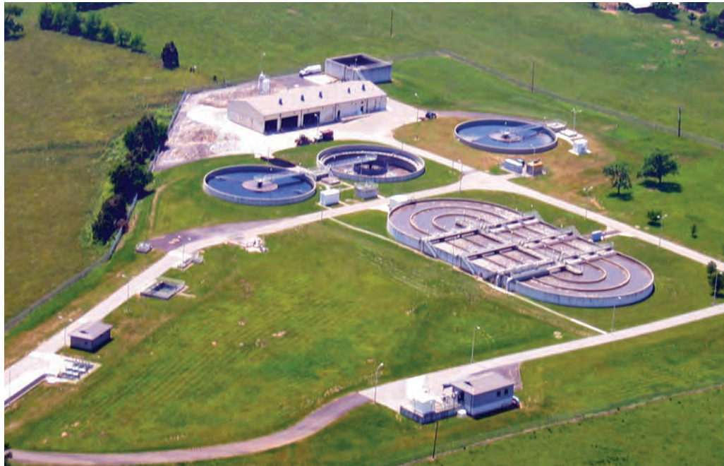
The City's wastewater treatment plant will double in capacity. Design has begun, and construction is planned to begin in early 2021. One clarifier pool (the round basin to the right) is already in place. The new facilities will be in the grassy and tree-lined section below it. The expansion will mirror the oval shaped oxidation ditch and add one additional clarifier as well as upgrade current pumps and electronic controls.
