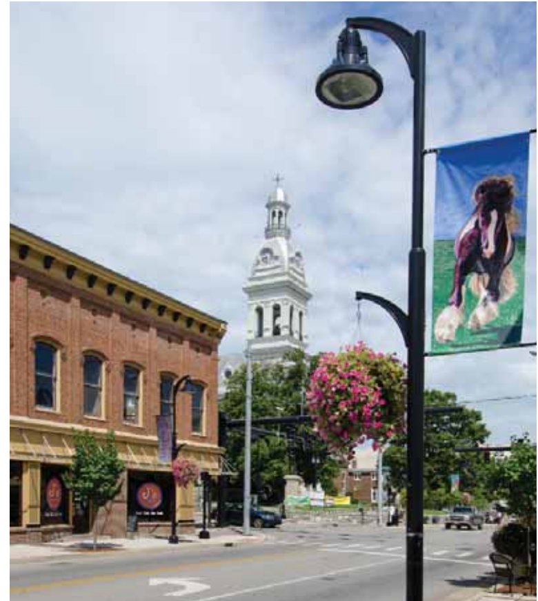
Phase II of the Streetscape project includes adding mast arms for traffic signals and removing the remaining wires that cross Main Street.
