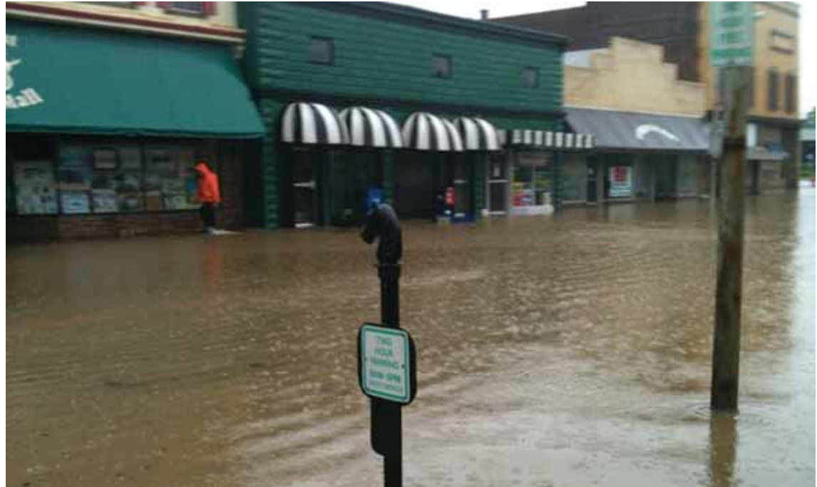
Flooding on Main Street will be resolved once the new dam is built south of the aquatic center in Riney-B Park.
